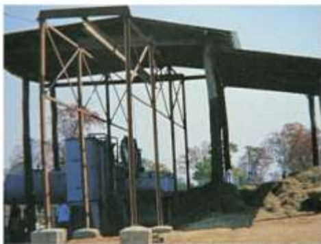
A Modern Field Still designed and fabricated by Eisseric of France and located in Nepal.
